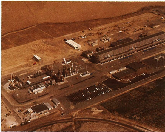
Union Carbide Corporation (UCC) funded the now operational silicon refinement production plant with 1200 MT/year capacity. DOE/FSA-sponsored efforts were prominent in the UCC process research and development.
