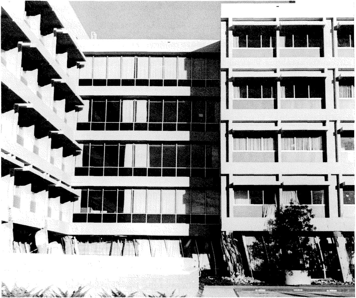
Figure 8.4 West elevation of the Olive View Hospital. The failure of this major new building and the collapse of the neighboring Psychiatric Day-Care Center show the need for improvement of seismic provisions in modern building codes.
