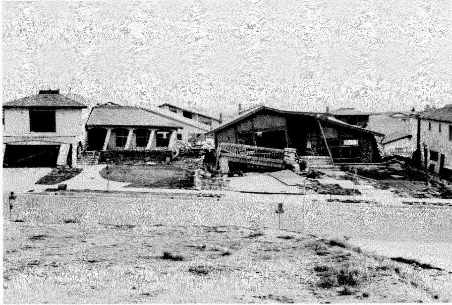
Figure 3.182 Two of the most severely damaged split-level houses on Almetz Street.
