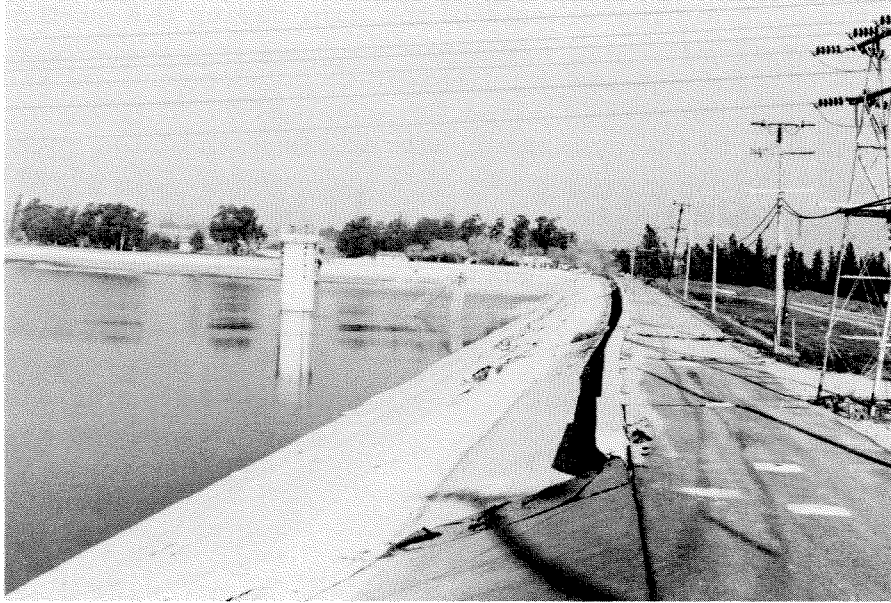
Figure 4.5 Downstream displacement of upper San Fernando Dam, looking east. Picture taken 21 February 1971.
