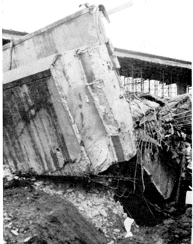
Figure 6.7 Seating detail of the western end of collapsed overcrossing, Golden State-Antelope Valley freeway interchange.
