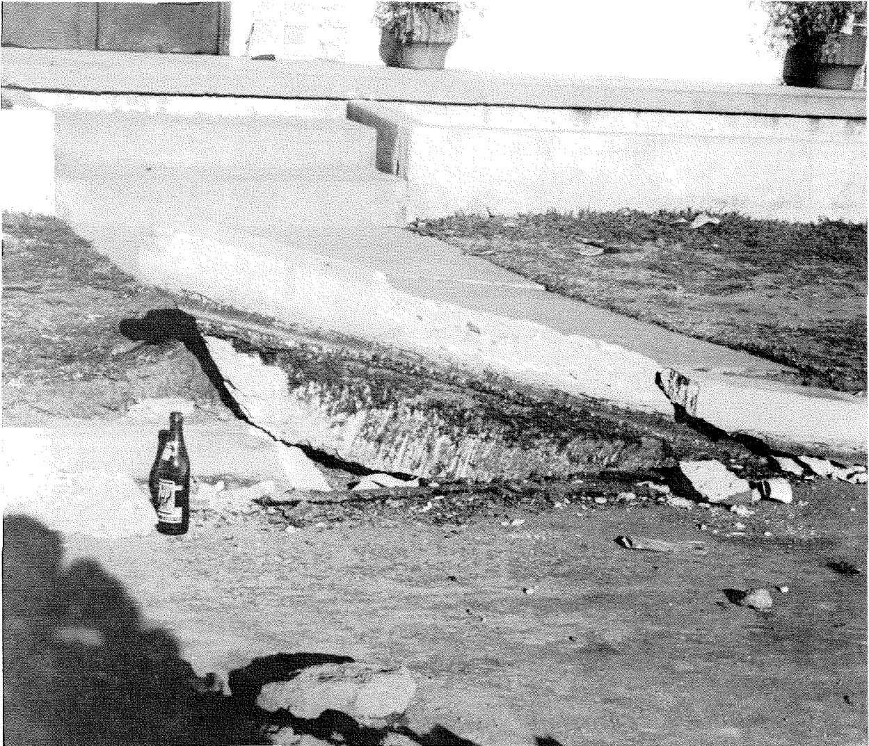
Figure 5.29 Shattered curb on northeast side of Glenoaks Boulevard about one block southeast of Hubbard Street. This approximately 18" of displacement of curb reflects the compressive deformation of the soil along this street where numerous gas line failures occurred.
