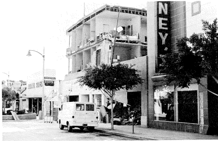
Figure 3.172 This building was hazardous not only to its occupants but also to the occupants of adjacent buildings and to passersby on the street.
