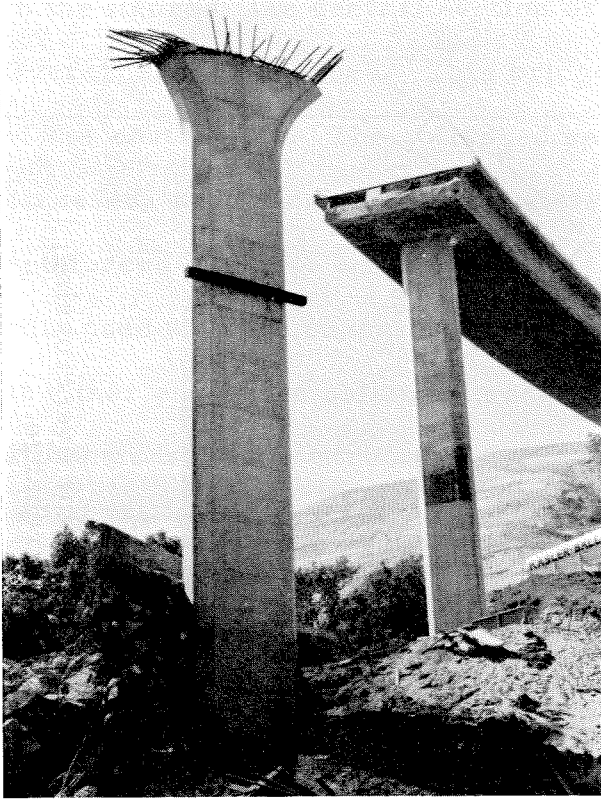
Figure 6.6 Western support for the collapsed overcrossing spans, Golden State-Antelope Valley freeway interchange.
