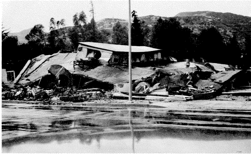
Figure 3.4 This old masonry building at Olive View Hospital, adjacent to the heating plant of the previous figure, was not designed to withstand earthquake loadings.
