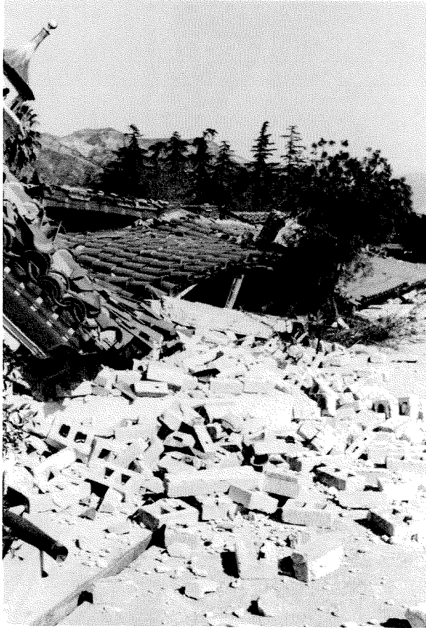
Figure 3.169 Collapsed old building at Olive View Hospital.
