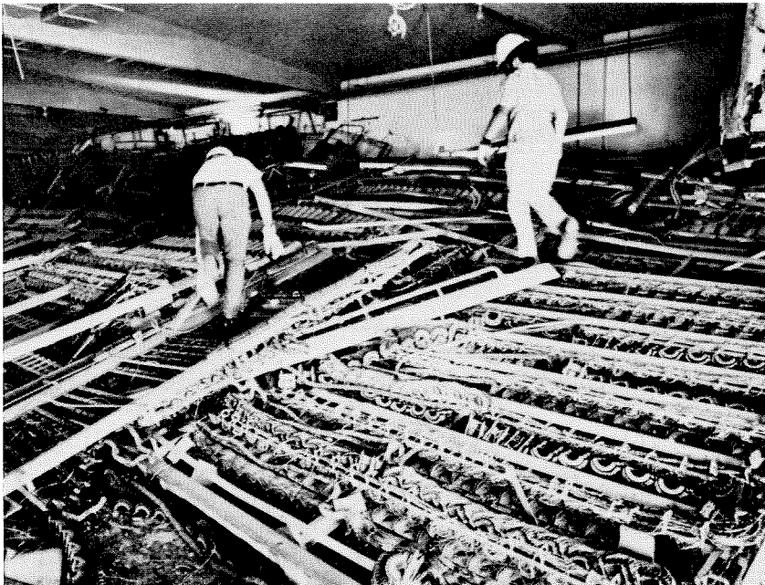
Figure 5.37 Interior of damaged General Telephone switching facility at Polk Street and Borden Avenue.
