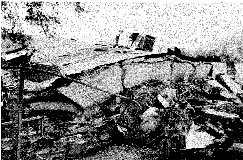
Figure 8.3 Old buildings at the Veterans Hospital. The greatest hazard to human life in California earthquakes comes from the older buildings, built before earthquake-resistant design provisions were incorporated in the building codes.
