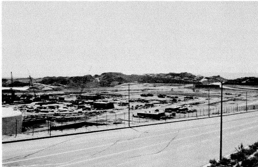
Figure 7.2 View looking southeast across Balboa Blvd. with the underground reservoir site in the background. Cracks in the Balboa Blvd. asphalt surface developed during the earthquake.
