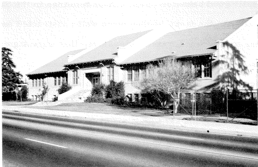
Figure 3.167 Morningside School at Maclay and Fifth Streets in San Fernando city. This 1915 building had been strengthened recently to make it satisfy the requirements of the building code for earthquake resistant design.
