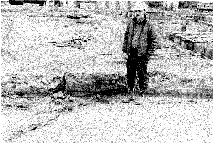
Figure 7.6 Cracks in access road to large water tank. In right-hand background is the control building which settled several inches; to the left is the steel frame chemical building which was damaged by excessive vibrations (cross-bracing failed).
