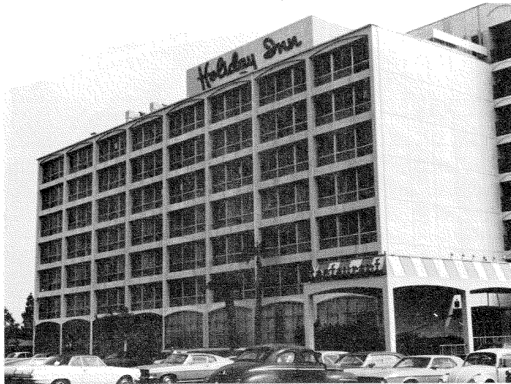
Figure 3.159 North elevation of Holiday Inn. This building is located at the intersection of Roscoe Blvd. and Orion St. six miles south of Balboa Blvd. Water Treatment Plant. Motion recorded on the ground floor had a peak acceleration of 27%g and motion recorded on the penthouse floor had a peak acceleration of 40%g.
