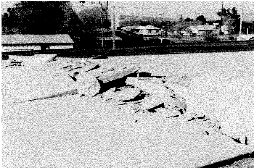
Figure 6.80 Shortening of freeway pavement caused by faulting. Foothill freeway near Maclay Street.
