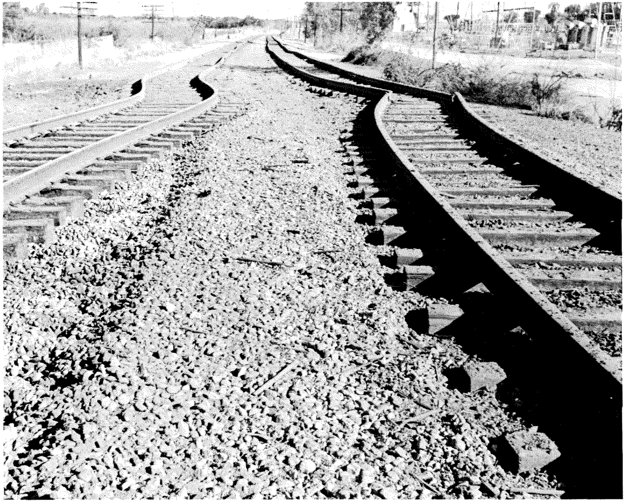
Figure 4. 15 The Southern Pacific Railroad tracks just south of the San Fernando Juvenile Facility at the east end show evidence of substantial ground movement.
