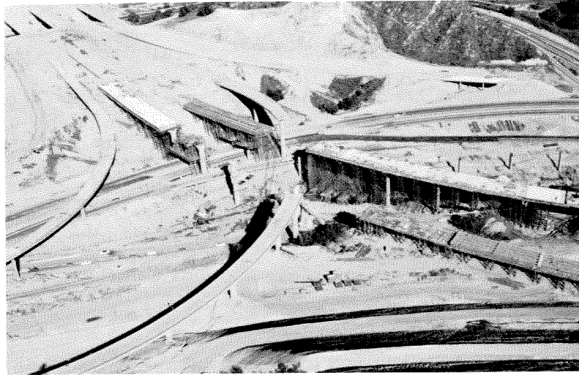
Figure 6.3 Post-earthquake view, looking east, of the Golden State-Antelope Valley freeway interchange.
