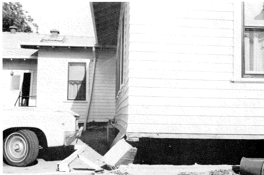
Figure 3.9 Old wooden building moved to the right and nearly fell from its concrete support props, Olive View Hospital.
