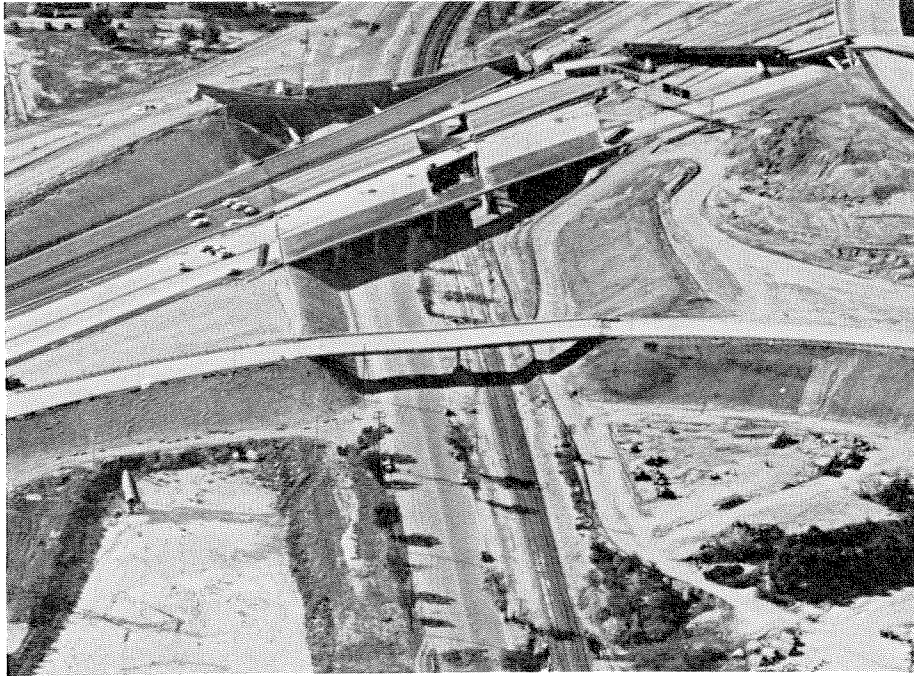
Figure 6. 37b. Aerial view of the San Fernando Road overhead.
