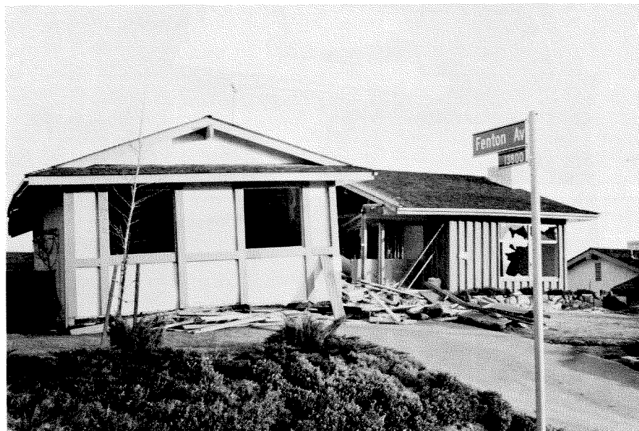
Figure 3.185 Garage walls collapsed from under the overhead bedroom of this split-level house on the corner of Fenton and Tyler.
