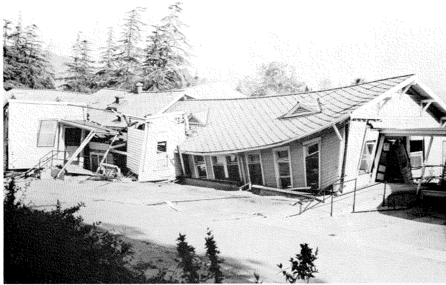
Figure 3.8 One of the more severely damaged old wooden buildings at the Olive View Hospital.
