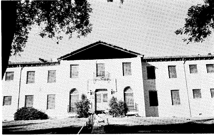
Figure 3.56 Nurses' Quarters (Bldg. 12) at the Veterans Hospital, as seen from the southwest. The gable wall fell in front of the entrance.
