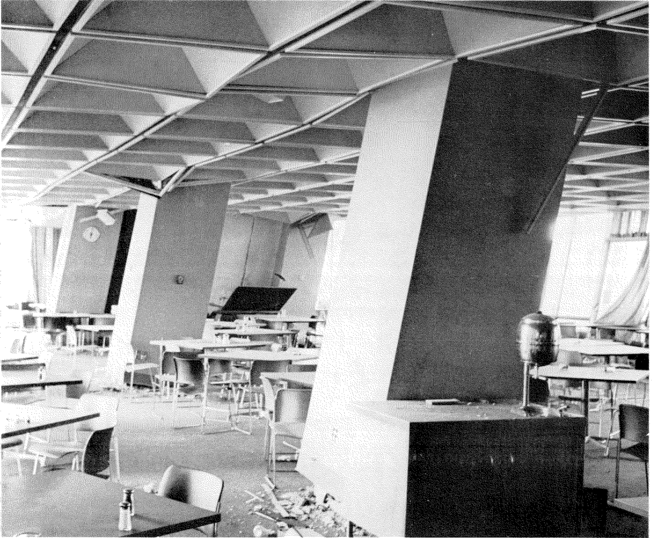
Figure 3.28 Cafeteria in Olive View Hospital.
