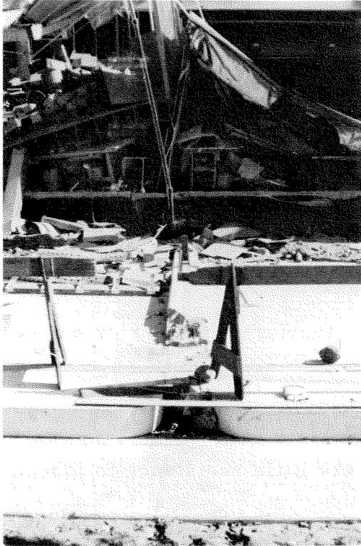
Figure 3.120 Collapsed tilt-up slabs showing the 12 in x 12 in column. Vector Electronics Building.
