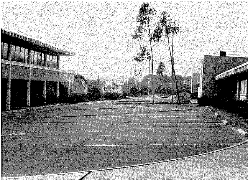
Figure 3.93 Interior courtyard looking west past collapsed wing of main building. Numerous cracks are visible in the asphalt parking area. San Fernando Juvenile Facility.
