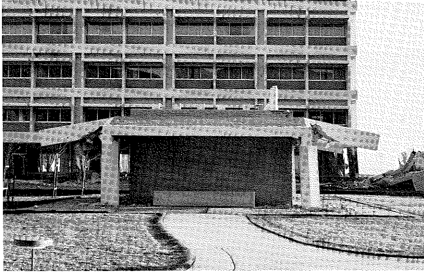
Figure 3.33 Exhaust pavilion to the north of the main building of the Olive View Hospital. The overhangs were originally horizontal. The cantilevered canopy was supported on four columns and is independent of the exhaust structure.
