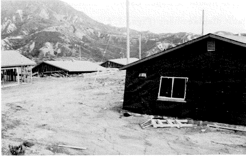
Figure 3.189 Heavily damaged and collapsed residential houses under construction, east of Veterans Administration Hospital.
