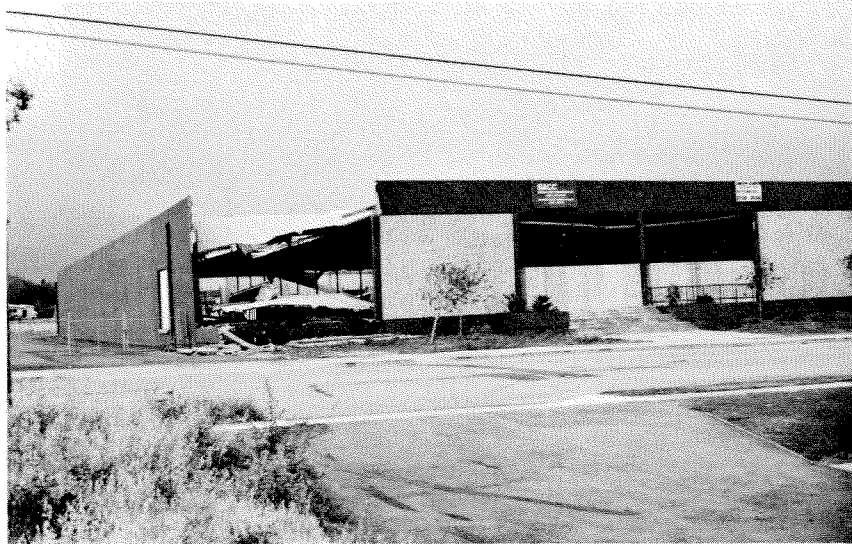
Figure 3.143 Collapse of a corner section in a new building at 12880 Bradley Avenue. The roof-to-wall connections failed at both the front and rear walls.
