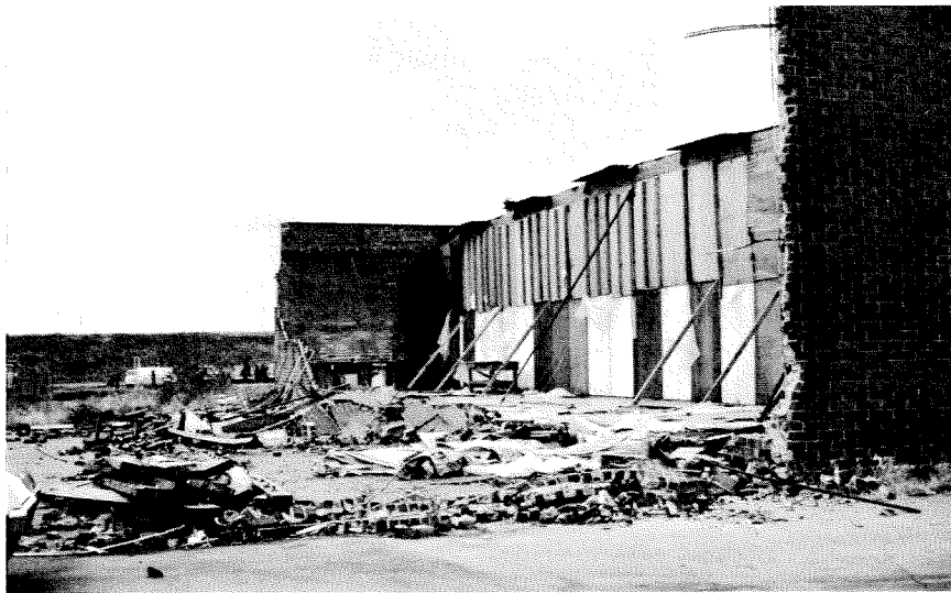
Figure 3.128 Collapse of brick wall (southeast wall). Bell Metrics Building.
