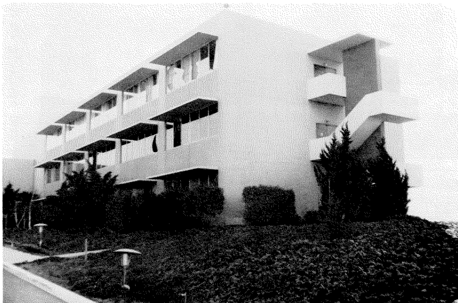
Figure 3.106 Three-story wing. Pacoima Lutheran Hospital, looking east.
