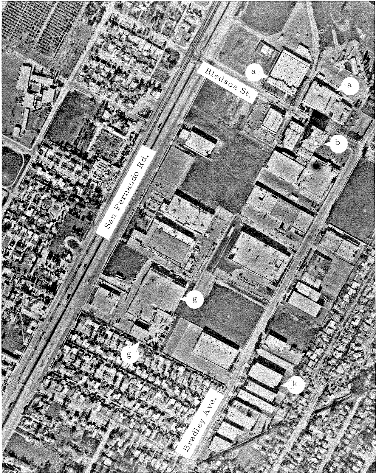
Figure 3.129 Roof collapses on tilt-up factory buildings. The identification letters refer to the list of buildings given in the text.
