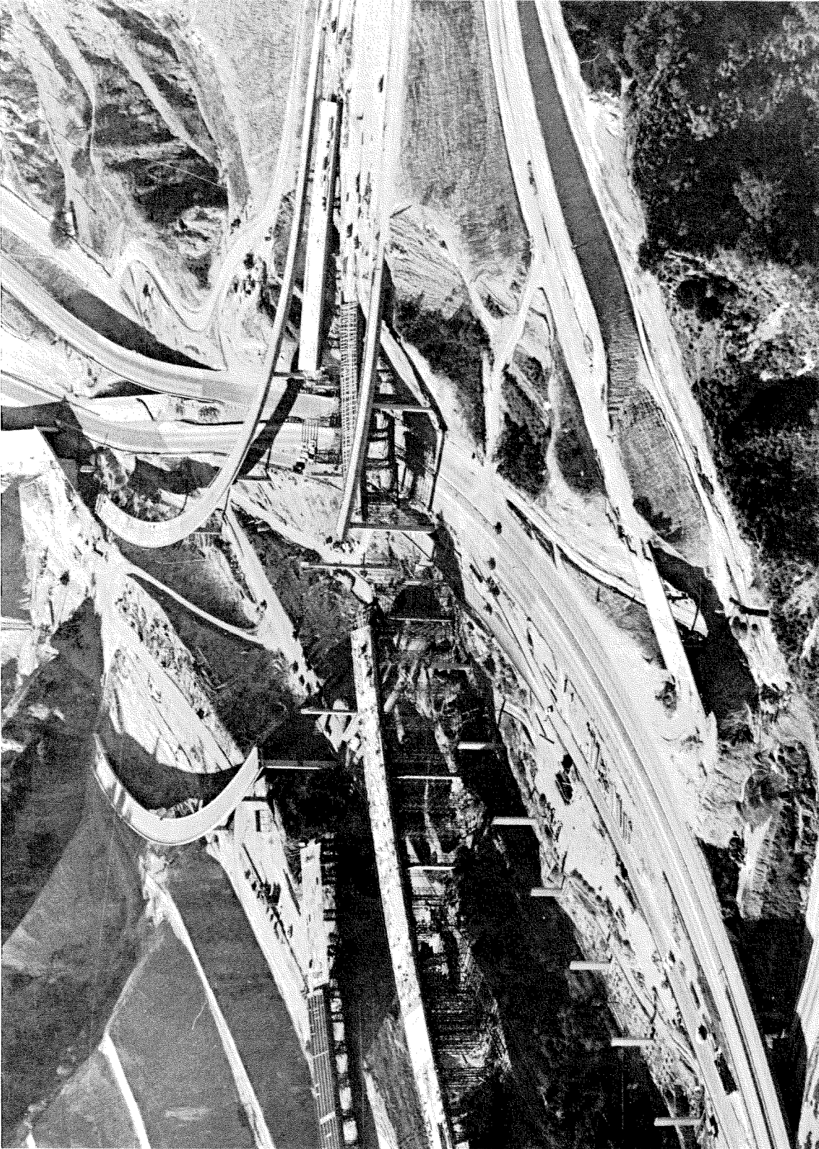
Figure 6.2 Post-earthquake view, looking west, of the Golden State-Antelope Valley freeway interchange. The center two spans of the highest overpass have collapsed. Photographed by Ralph Samuels
