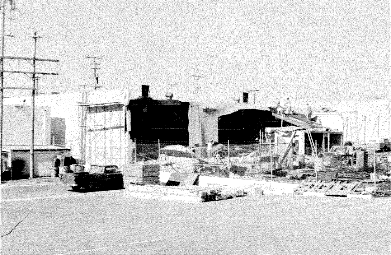
Figure 3.127 Collapse of concrete block wall (northeast wall). M & L Machine and Stamping Company Building.
