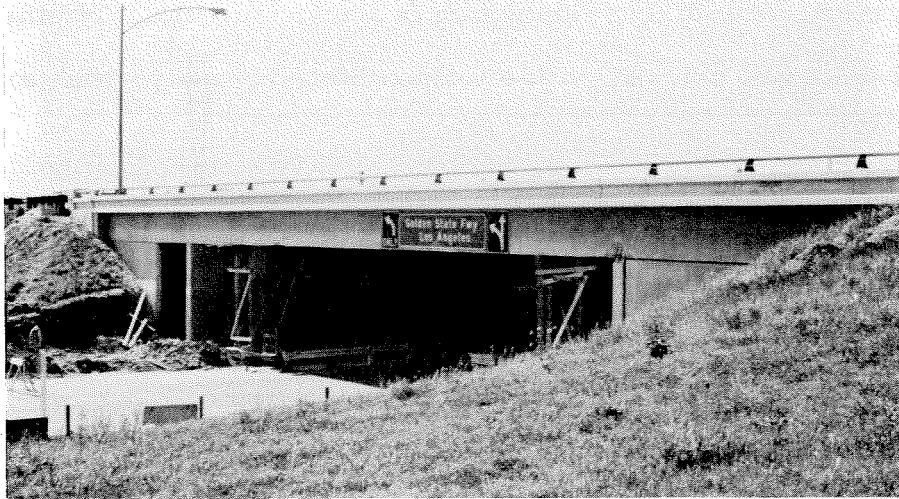
Figure 6.81 Roxford Street undercrossing, looking south, Golden State freeway.
