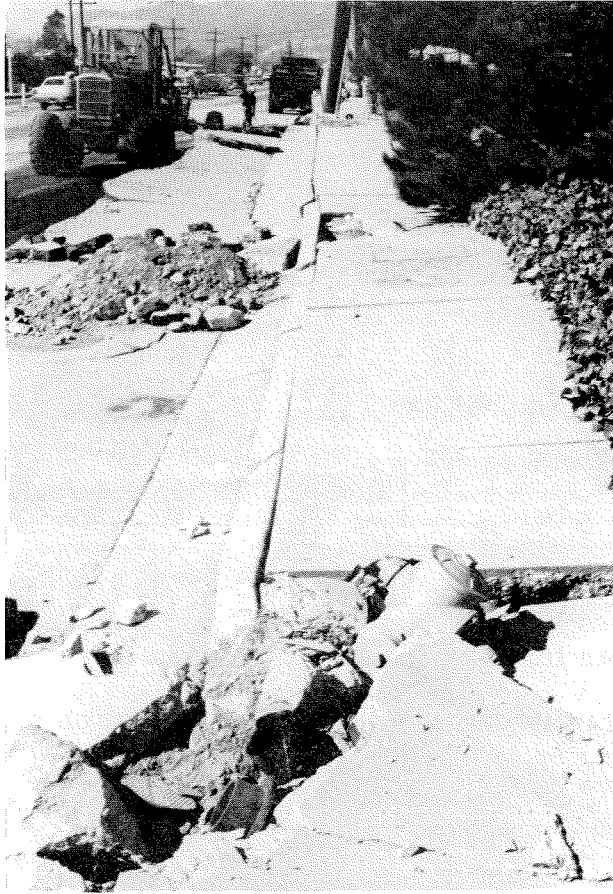
Figure 5.35 Fire hydrant broken by ground movements, Sylmar area.
