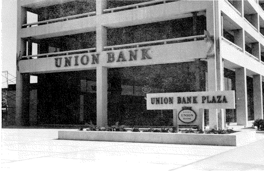
Figure 3.149 The cracks in the reinforced concrete frame were filled with epoxy, Union Bank building, Sherman Oaks.
