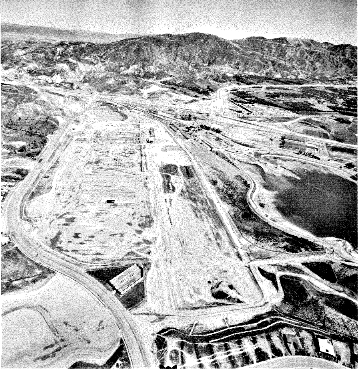
Figure 4.8 Aerial photograph of Jensen Treatment Plant, looking north, on 11 February 1971. Slope movement has occurred on hill to west. Upper Van Norman Reservoir is to the right.
