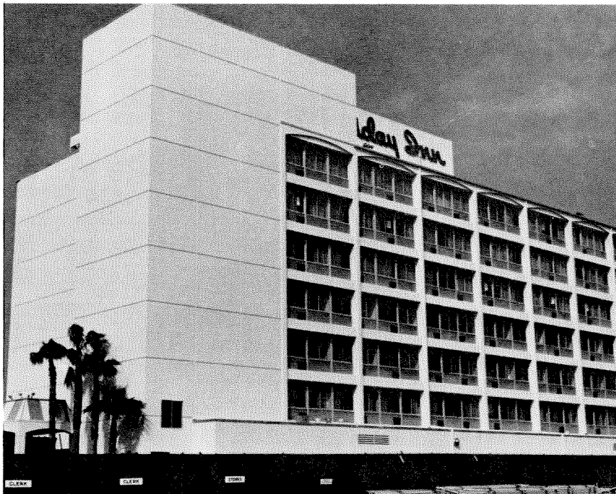
Figure 3.162 South elevation of Holiday Inn. The concrete frame underwent some cracking which indicated strains beyond the yield point.
