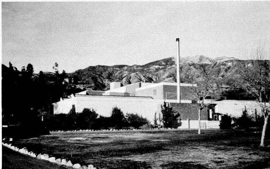
Figure 3.7 New laboratory building at Olive View Hospital received only minor damage.
