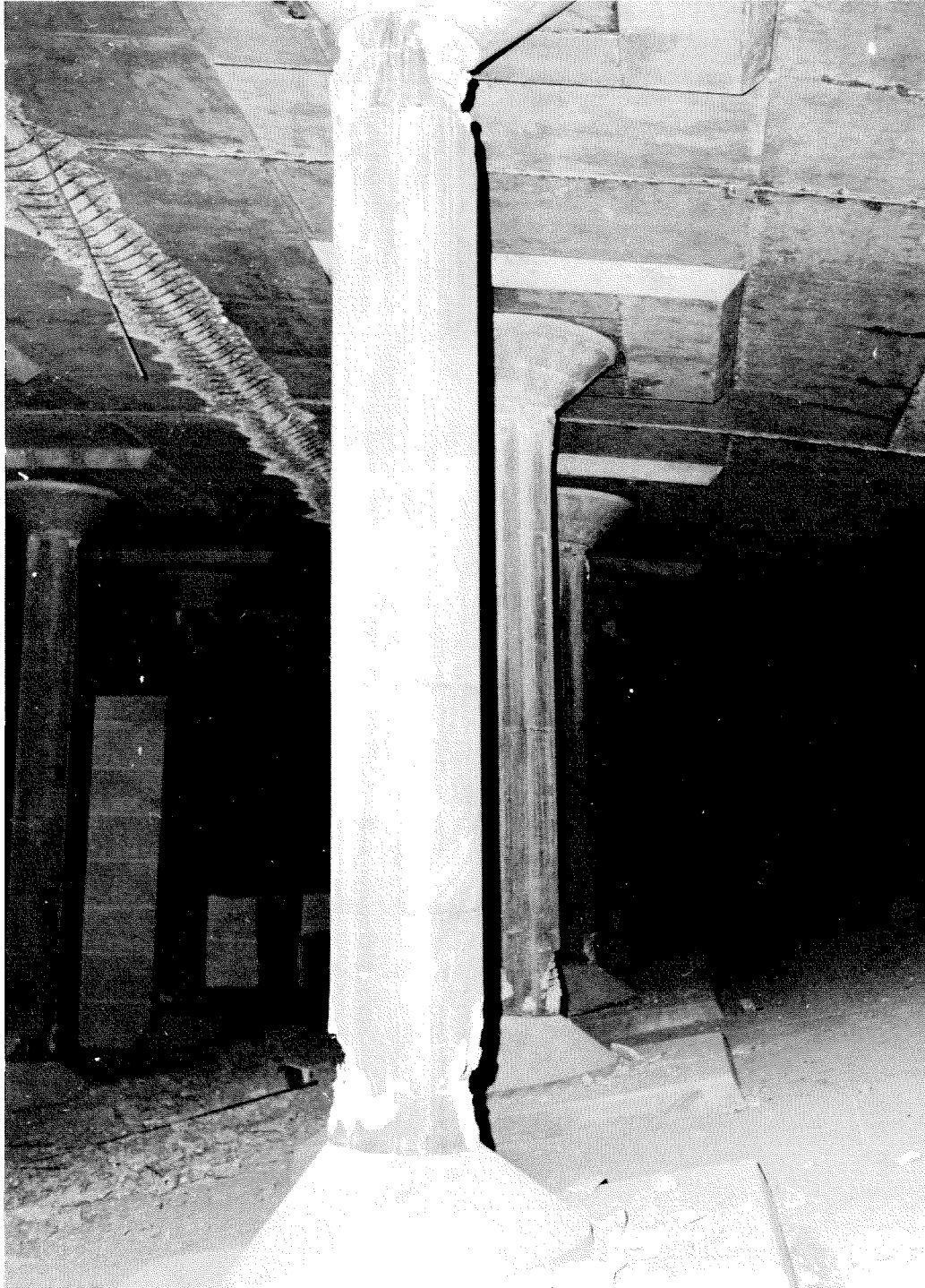
Figure 7.11 Interior view of reservoir showing typical column failures and a difference in elevation across roof slab damage along the construction joint. (MWD photograph).
