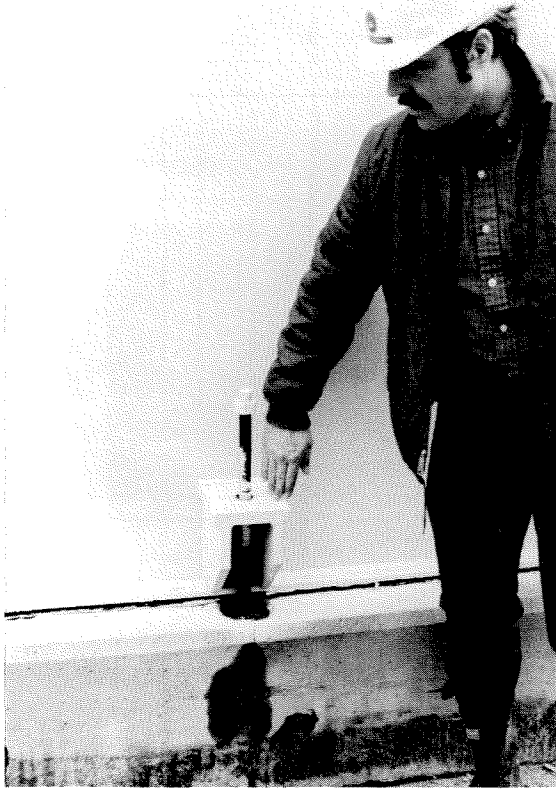
Figure 7.20 Anchor bolt pulled up on west side of tank.
