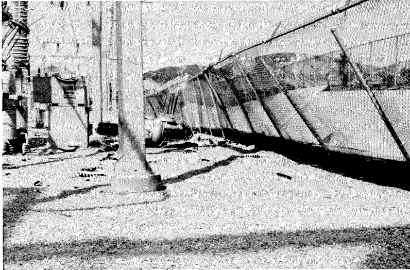
Figure 4.13 Ground displacements along fence and drainage channel at northeast boundary of Sylmar Converter Station. The settlement of the station in foreground with respect to the concrete lining of the channel is apparent.
