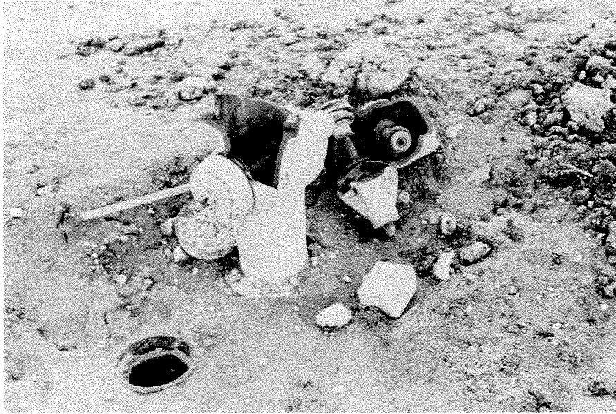
Figure 7.22 Cast iron water hydrant east of the settling basins was found shattered after the earthquake. MWD treatment plant.
