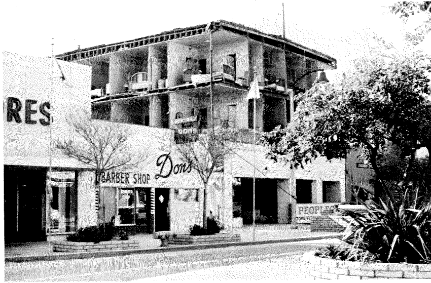
Figure 3.171 Brick walls of old building in San Fernando city collapsed leaving floors supported on interior wood and plaster partitions.
