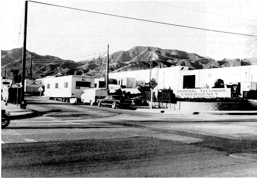
Figure 5. 36 General Telephone switching facility at Polk Street and Borden Avenue.
