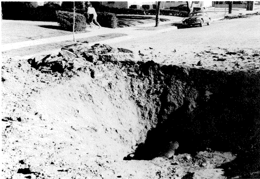
Figure 5.31 Crater from ruptured gas main on Glenoaks Boulevard. The 16 in diameter line has already been repaired.
