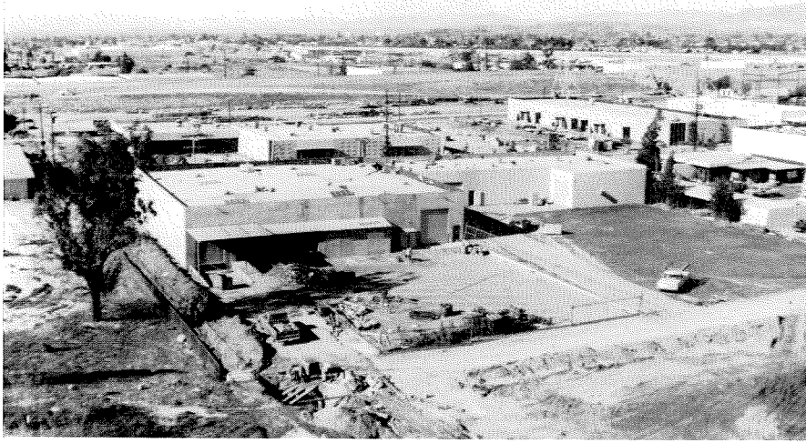
Figure 3.114 San Fernando Industrial Park. Omneco and Cosmic Plastic Buildings in the foreground. Permanent ground displacements have forced these buildings together causing serious structural damage.
