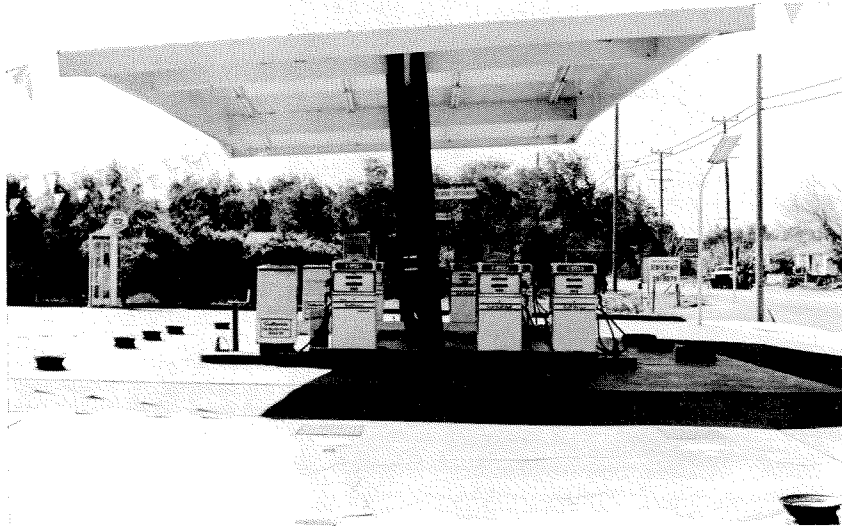
Figure 7.29 Pergola at gasoline station at the corner of Glenoaks Boulevard and Roxton Avenue yielded at base. The supporting members are steel pipe columns.
