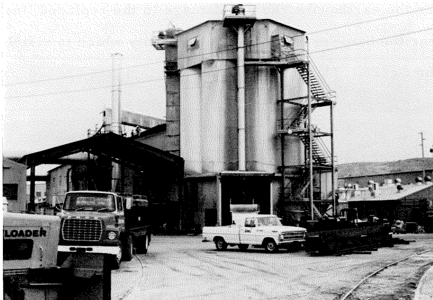
Figure 7.47 Thatcher Glass Factory between Newhall and Saugus. This large cluster of storage bins had its first-story supports damaged. The bins are supported on steel columns with I-beam bracing. The bracing was overloaded and underwent permanent deformations.
