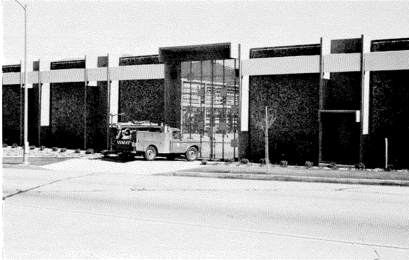
Figure 7.24 Balboa Blvd. switchyard is surrounded by decorative cantilevered walls, presumably designed according to the requirements of the building code.
