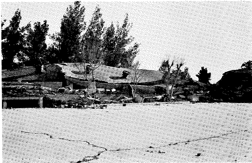
Figure 3.57 Collapsed Engineering and Shop Building at the Veterans Hospital.
