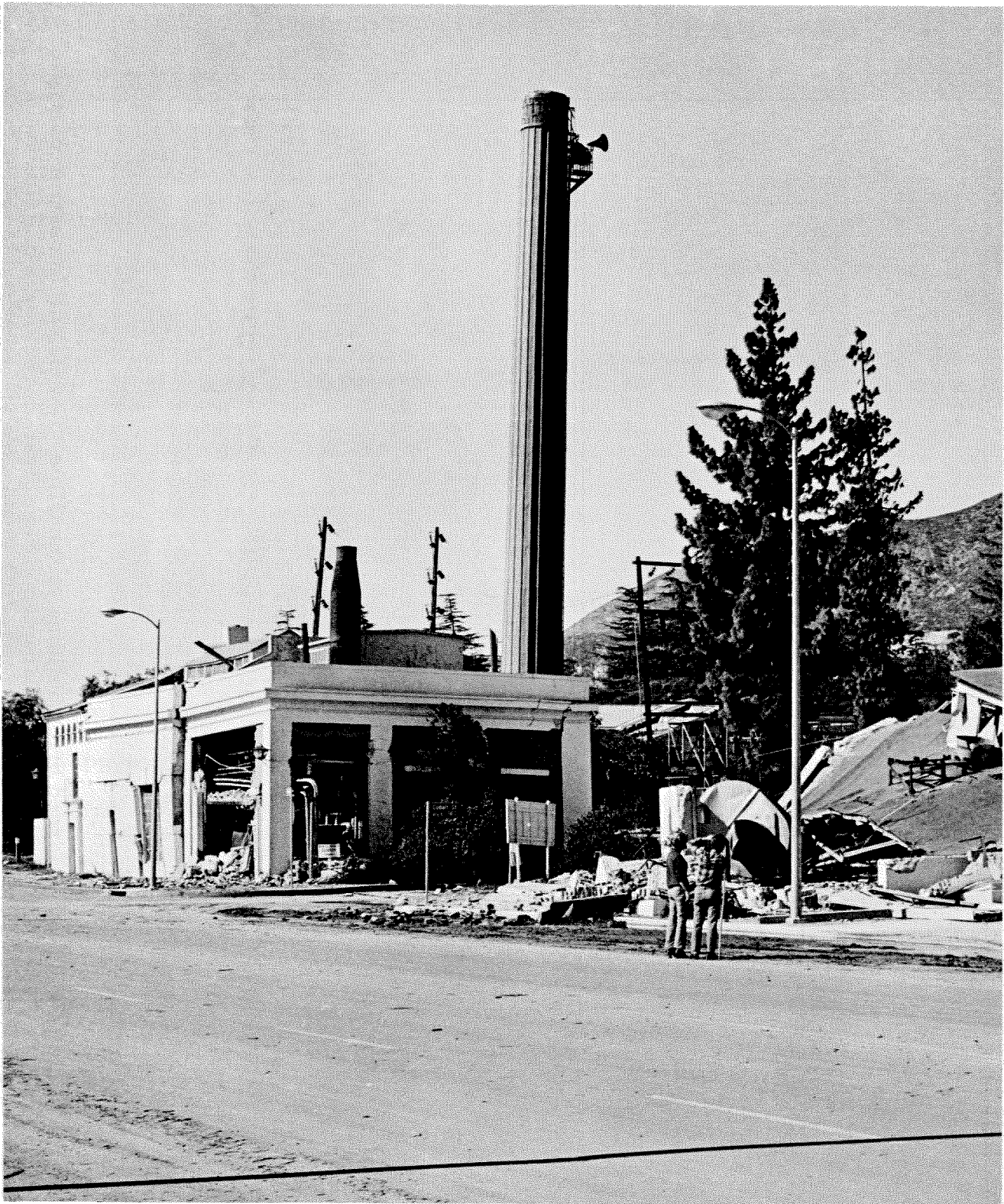
Figure 3.3 The old heating plant was severely damaged and the masonry building to the right collapsed at the Olive View Hospital. The concrete stack, which is leaning slightly, was removed shortly after the quake. Ralph Samuels photo.
