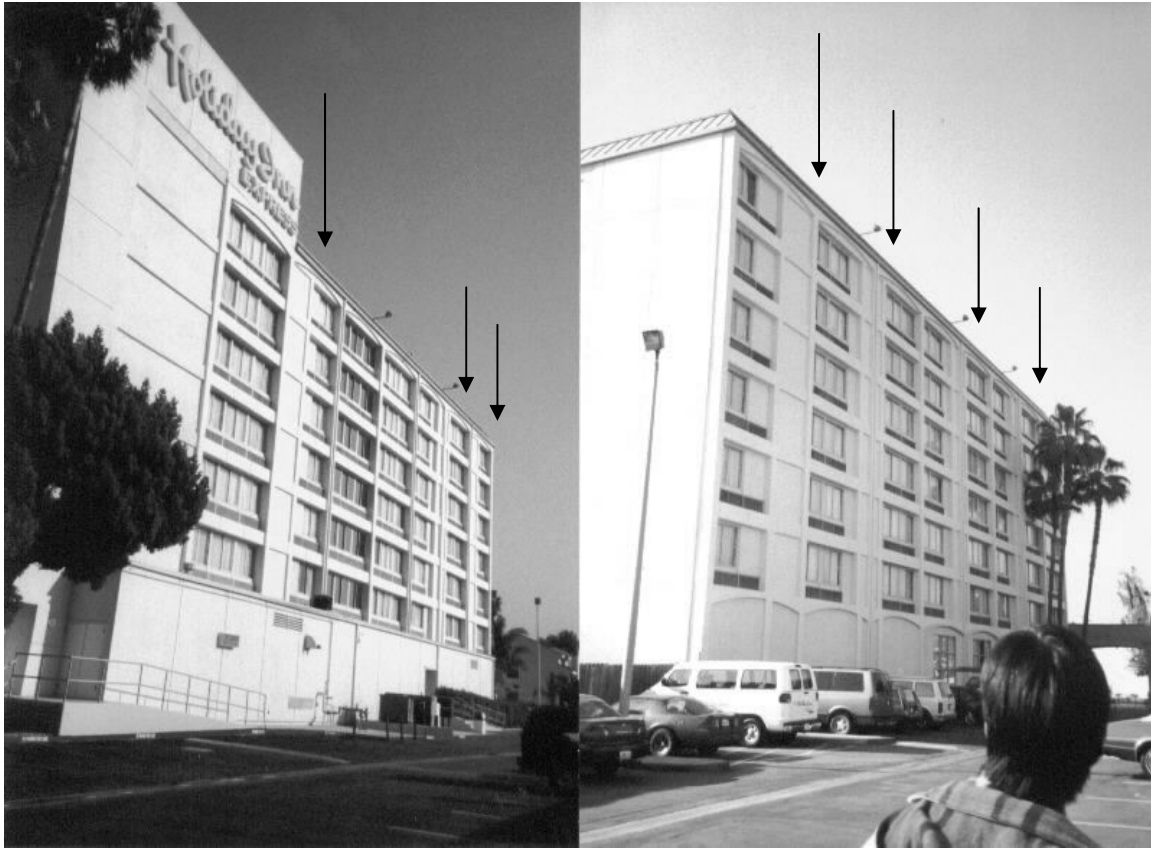
Figure 4-16. Shearwalls added to south (left) and north frames (right) after the 1994 Northridge earthquake. (Left: lines A-3, 7 and 8 from near to far. Right: lines D-8, 7, 5, and 3)
