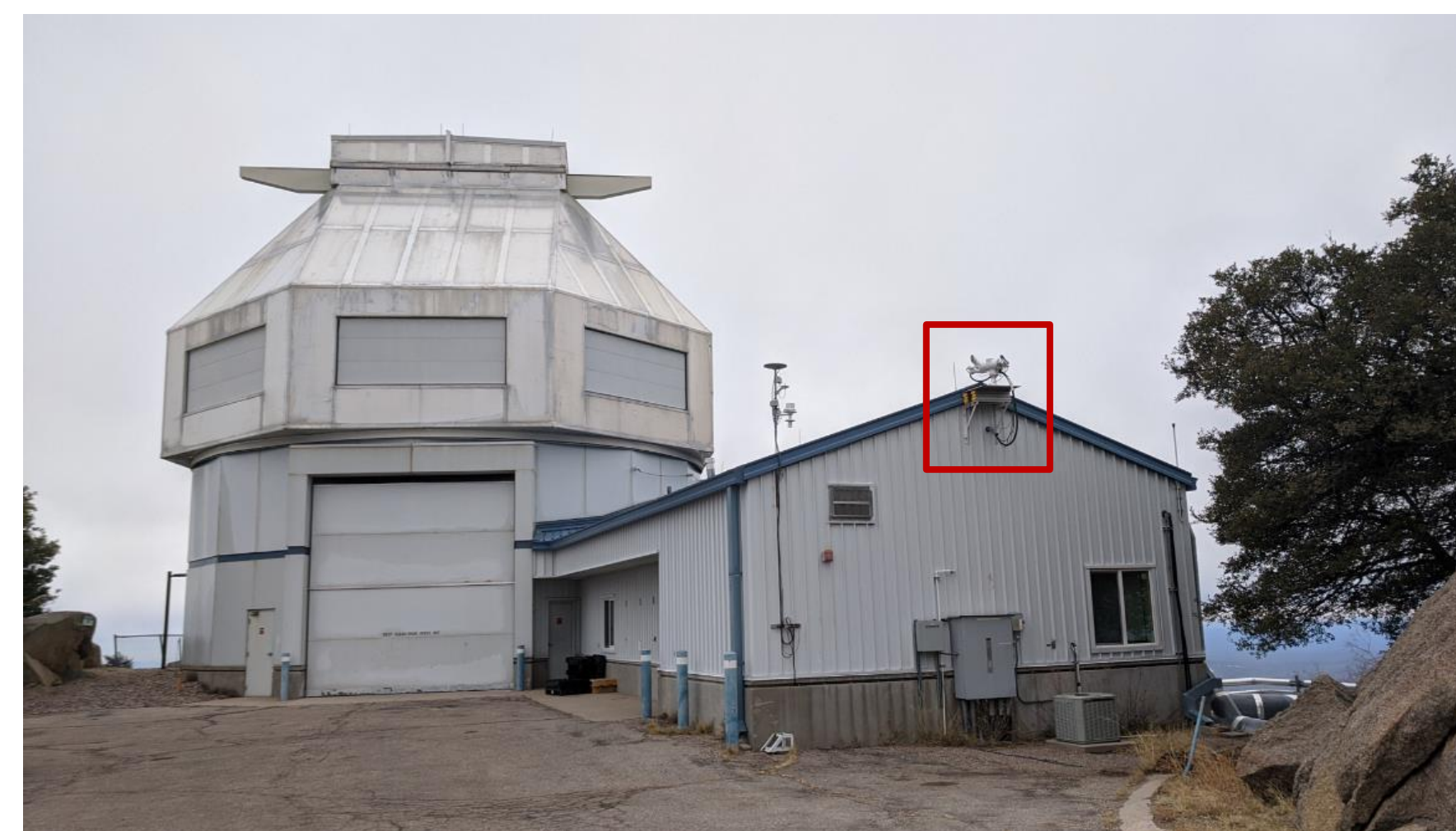
Fig. 2: The solar feed (red box) installed on the control building of the WIYN 3.5m. This location permits an unobstructed view of the sky above airmass 2 throughout the year and is accessible for periodic maintenance.
