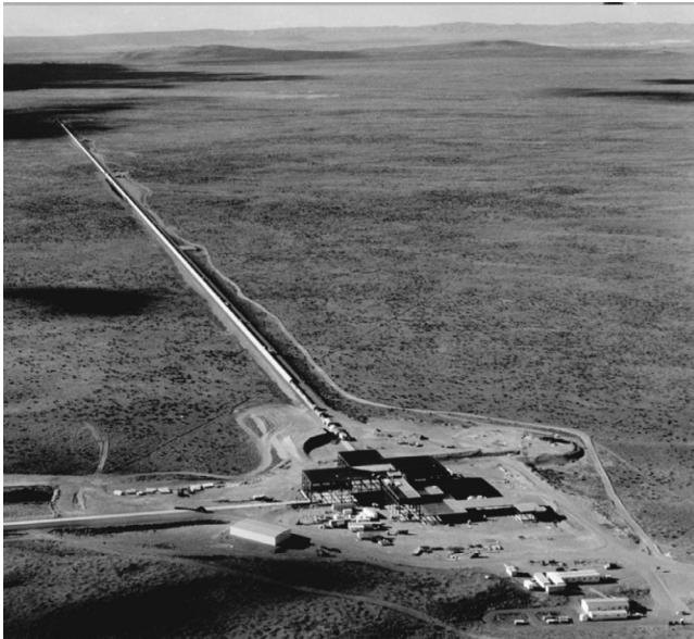
FIG. 1. Aerial view of the LIGO site at Richland, Washington.
