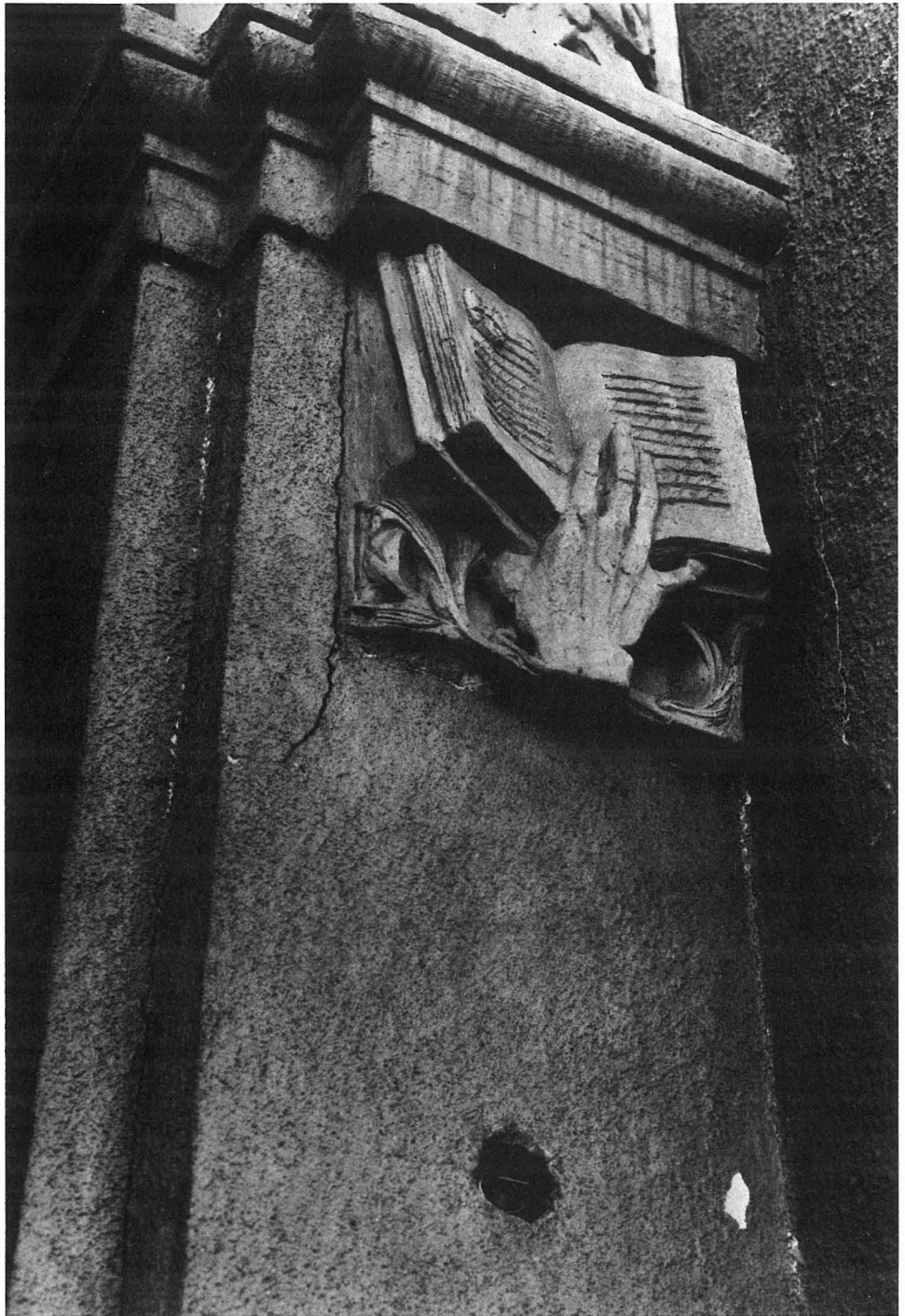
One of Calder's corbels, a haunting hand on an open book, is surrounded by earthquake cracks.
