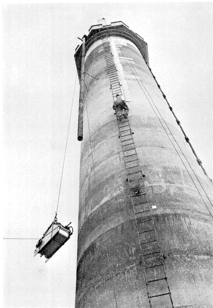
Fig. 12. Vibration Exciter Unit Being Hoisted to Top of Tower
