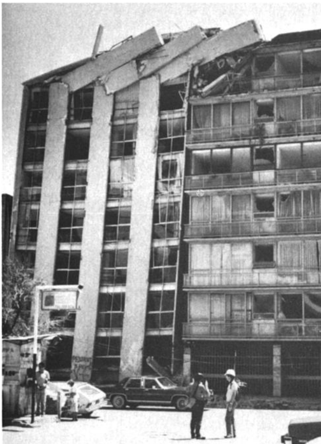
Fig. 7. Impact damage.
