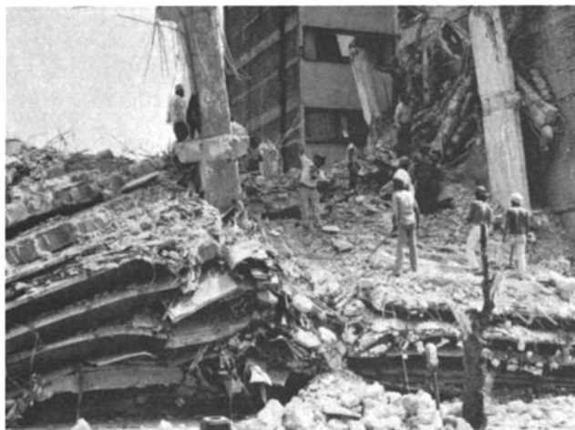
Fig. 3. Flat plate construction.
