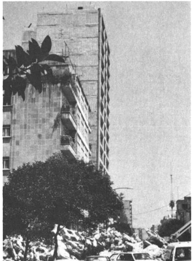
Fig. 8. Foundation failure.
