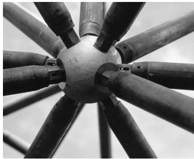
Figure 9. Node of bolted steel primary mirror support truss.
