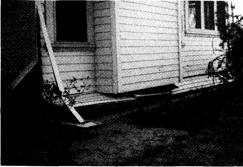
Figure 17. Failure of older wooden homes on unbraced foundations was evident in the San Fernando earthquake, and continues to be a common, preventable feature of California earthquakes in the areas of strong shaking.
