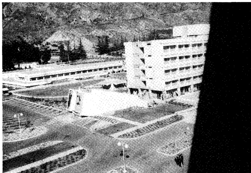
Figure 6. A portion of Olive View hospital as seen from a helicopter the afternoon of the earthquake. The stair tower in the foreground fell into the basement. The first floor of the two story Psychiatric Day Care Center collapsed in such a way as to leave the second story virtually intact.
