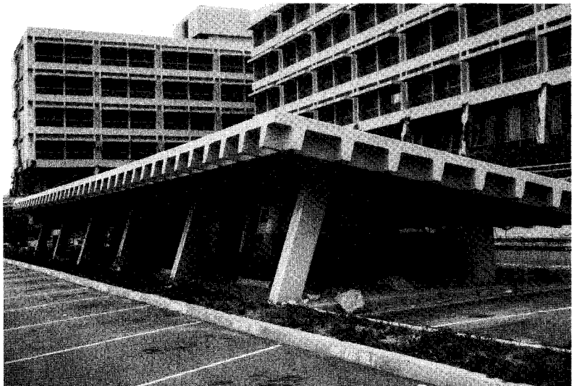
Figure 9. The collapsed pergola at the Olive View hospital destroyed the hospital's emergency vehicles. The stresses on the emergency services from the moderate-sized San Fernando earthquake pointed to the need for back-up facilities and careful planning in the event of a larger shock.
