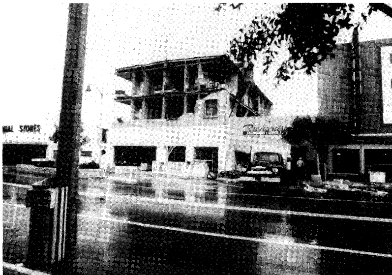
Figure 13. Failure of old buildings was an expectable feature of the San Fernando earthquake, accounting for nearly all of the casualties. This old brick building in downtown San Fernando showed the classic loss of exterior walls, while the partitions held up the remaining structure. Any occupants of the upper story bedrooms must have had an unforgettable experience.
