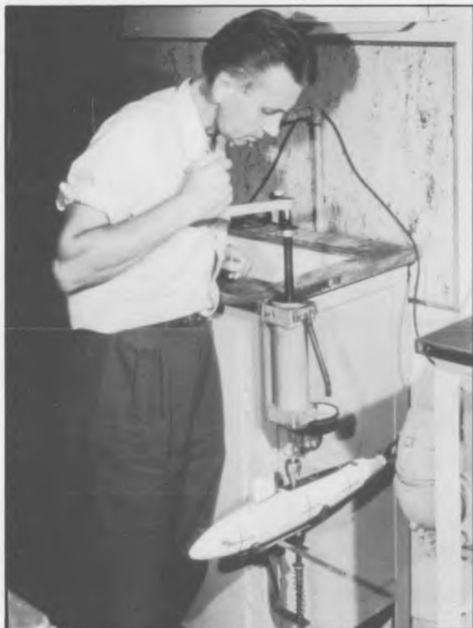
Fig. 3-5 Charging accumulator with metering pump.
